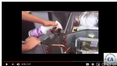
Leak Report Using Video
