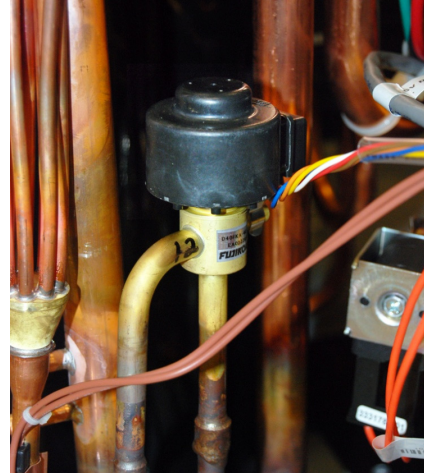
Fig. 1 – Electronic Expansion Valve (EXV)
