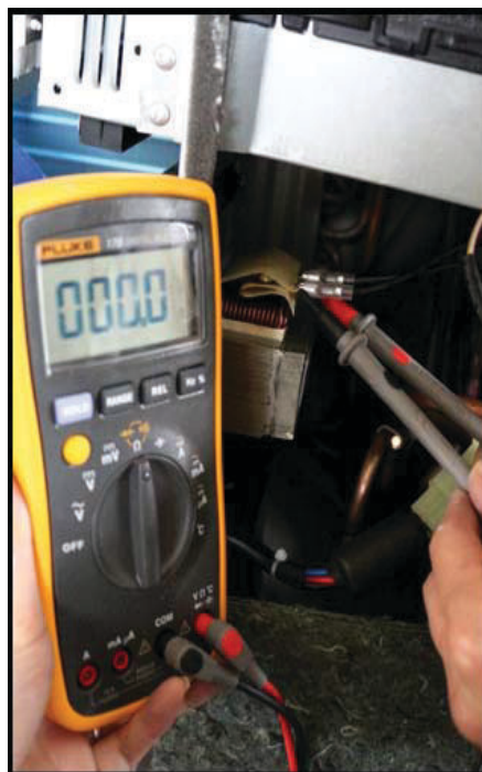
Fig. 24 —Test the Reactor resistance
