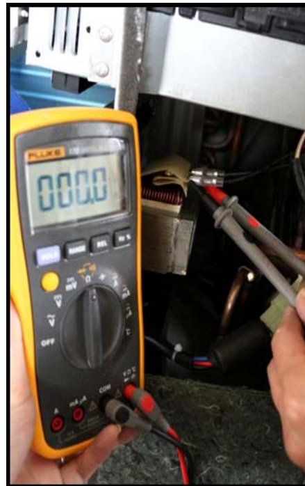
Fig. 24 – Test the Reactor Resistance
