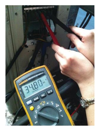
Fig. 43 —Test the DC voltage
